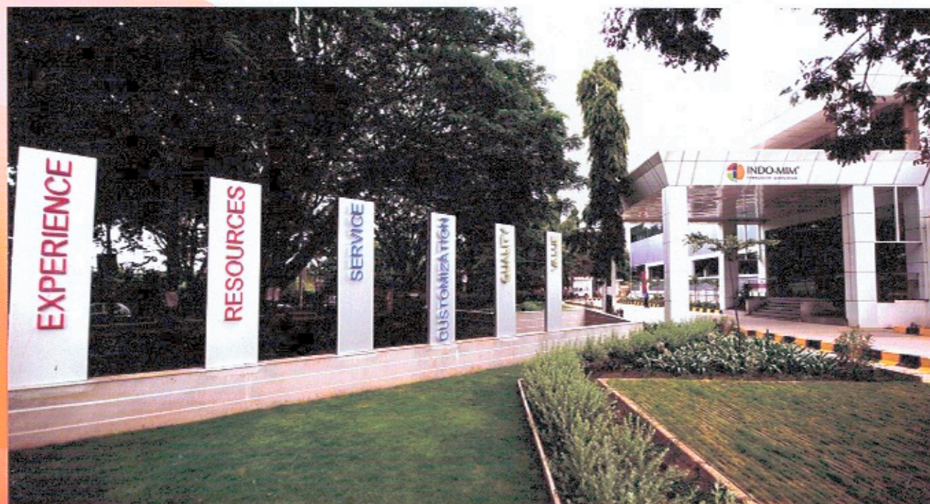
Doddaballapur Manufacturing & Finishing Facility, Bangalore
